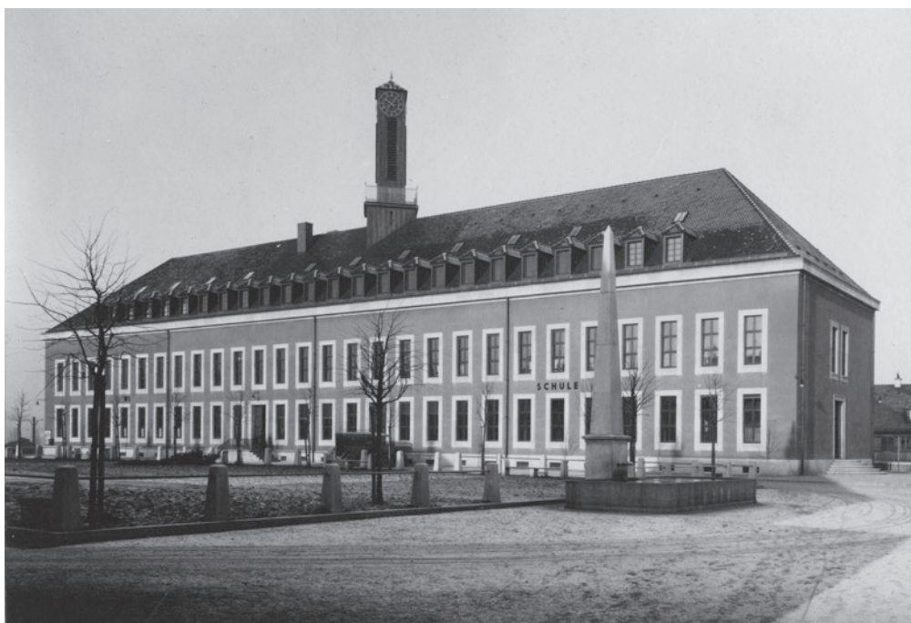
Hannes Meyer, the community building of the co-operative housing estate Freidorf, 1924, photo: Theodor Hoffmann
